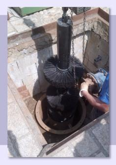
The winch can be placed close to the wellhead to allow the unit easy access into the well or borehole. Following the introduction of the appropriate **BoreSaver treatment**, the rig's specially designed brushes are lowered into the bore casing to the areas of contamination and then oscillated up and down to affect a brushing and surging motion. The brushes from the hydraulic rig remove encrustations and bacterial growth from casing walls/screens and out into the formation.
